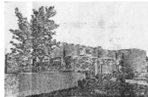
Old Western University (top), picturing Ward Hall and the Industrial Building, is shown on a postcard circa 1909. The Bryant-butler-Kitchen Nursing home (bottom) is one of three facilities in that approximate area today.
