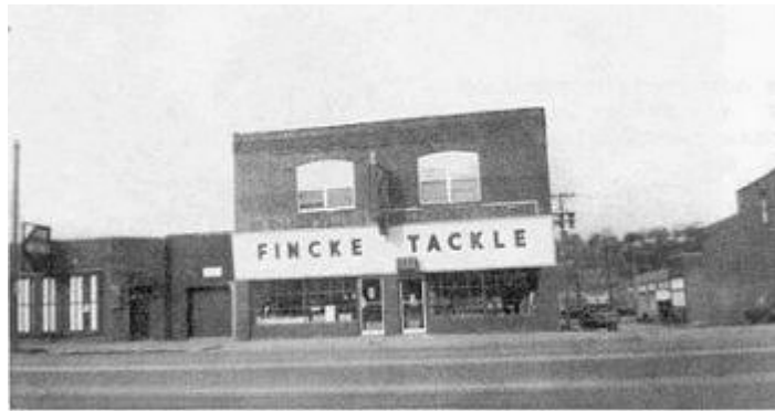
Chris W. Fincke built this building for his Feed, Hay and Grocery business at 726-728 Southwest Blvd. During the past 76 years, some member of the Fincke Family has been in business in this building. Julius Fincke, the Coal business for many years. Another son, Lou Fincke, the Hardware business. Now a grand-son has the Fincke Tackle Co.
