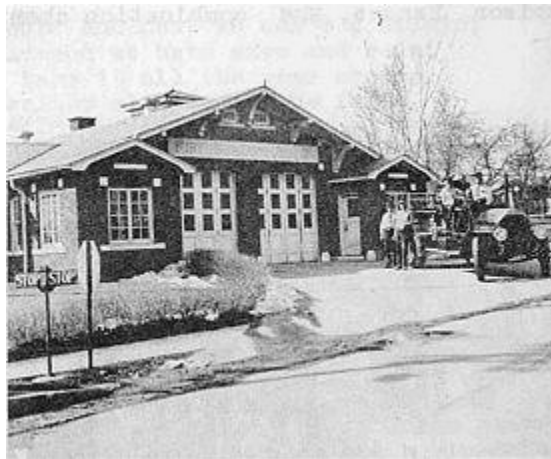
Kansas City, Kansas Fire Station No. 12
