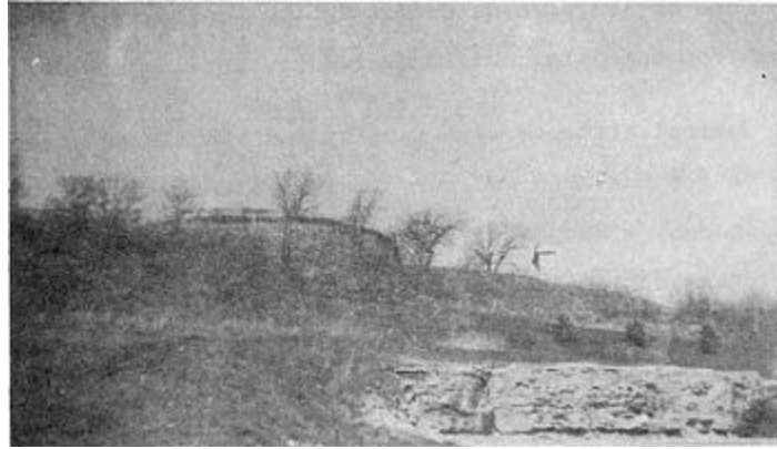
View of Retaining Wall from Rainbow Boulevard
