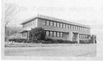
Frisco Office Building
