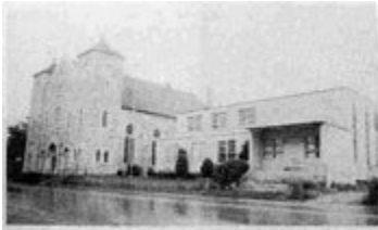
HOLY NAME CHURCH AND SCHOOL Southwest Blvd. And Iowa Street
